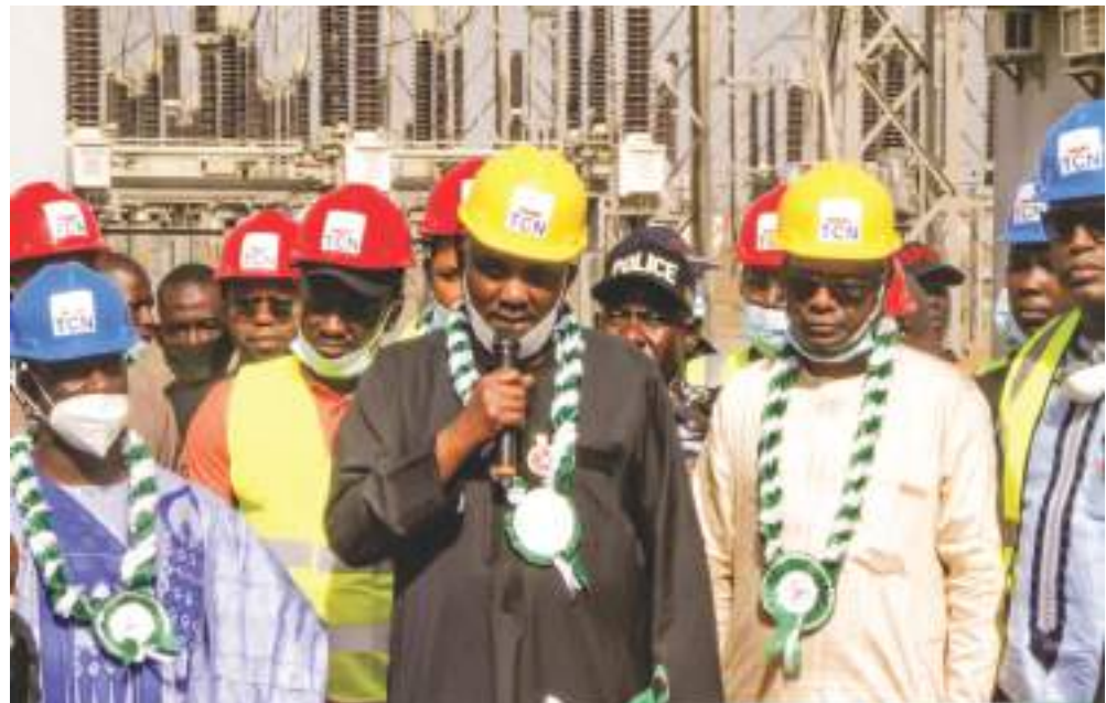
Middle Minister of Power, Engr Sale Mamman flanked on the right by Ag MD/CEO TCN Engr. Sule Abdulaziz during the commissioning of 150MVA Transformer in Kumbotso, Kano State
