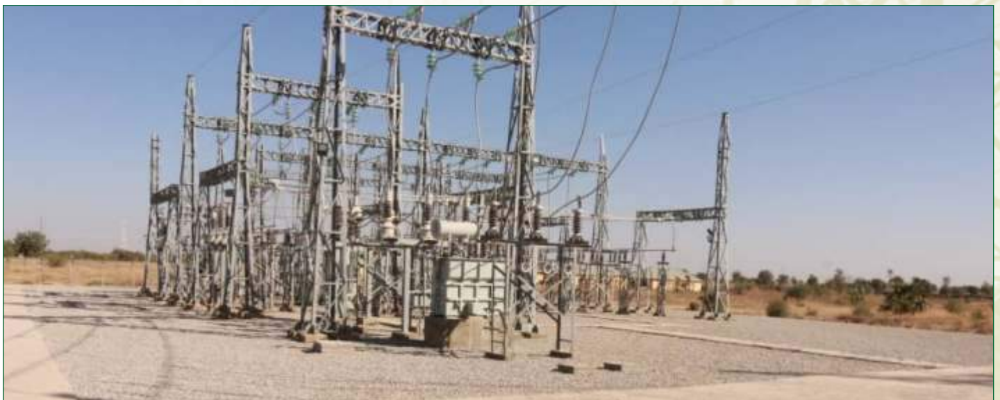
The brand new 30/40MVA, 132/33 Transmission Substation in Wudil
