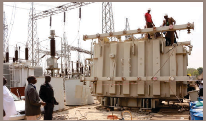
On-going repair works by TCN's engineers on a faulty 60MVA Power Transformer
