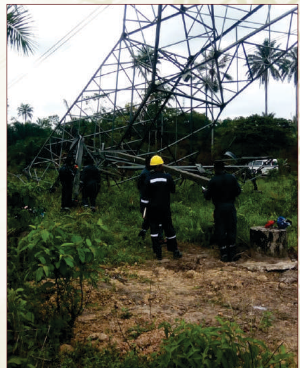
One of the vandalised tower
