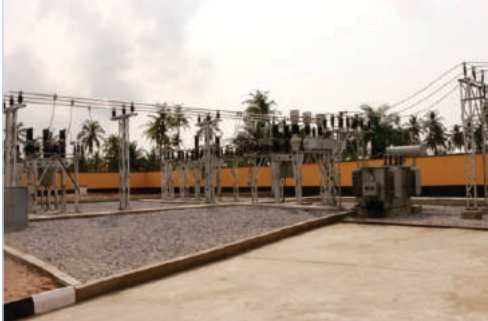
The new 132/33kV transmission substation at Ilashe, by TCN engineers
