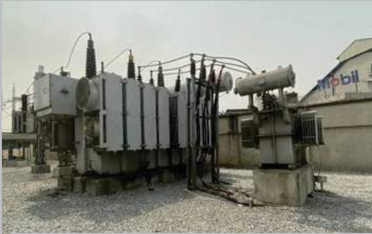
45MVA 132/33kV power transformer in Apapa 132/33kV Transmission Substation, Lagos State, commissioned Wednesday, 29th January, 2020
