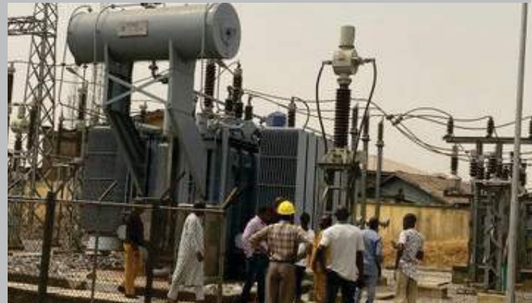
100MVA 132/33kV power transformer in Ogba 13233kV Transmission Substation, Lagos State, commissioned Wednesday, 8th January, 2020
