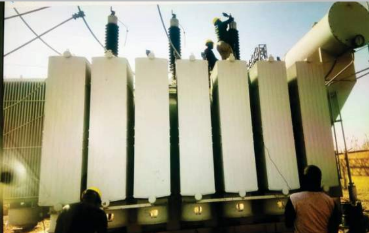
60MVA 132/33kV power transformer in Gusau Transmission Substation, Zamfara State, commissioned Thursday 23rd January 2020
