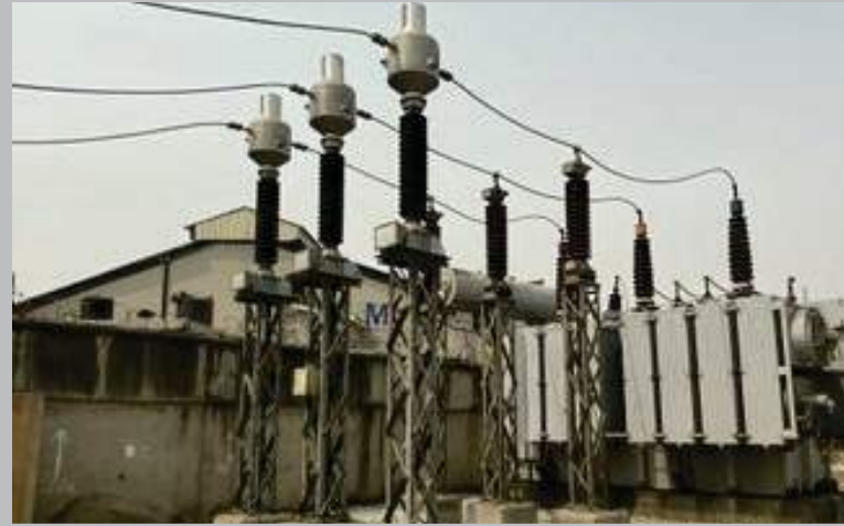
45MVA 132/33kV power transformer in Apapa 132/33kV Transmission Substation, Lagos State, commissioned Wednesday, 29th January, 2020
