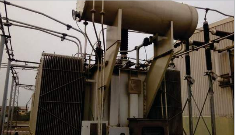
60MVA 132/33KV Transformer at Aja Transmission Substation, Lagos State, commissioned Monday, 27th January, 2020
