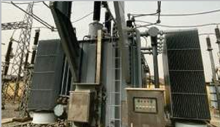
100MVA 132/33kV power transformer in Ogba 13233kV Transmission Substation, Lagos State, commissioned Wednesday, 8th January, 2020
