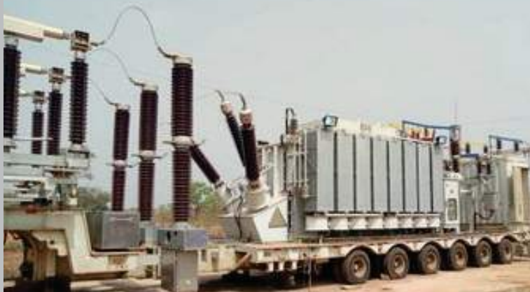
40MVA 132/33kV mobile power transformer installed in Etsako Transmission Substation, Edo State, commissioned Thursday, 9th January 2020
