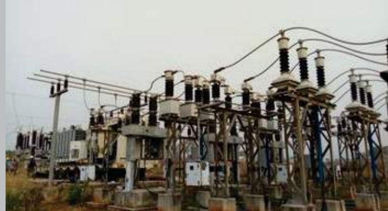
40MVA 132/33kV mobile power transformer installed in Etsako Transmission Substation, Edo State, commissioned Thursday, 9th January 2020
