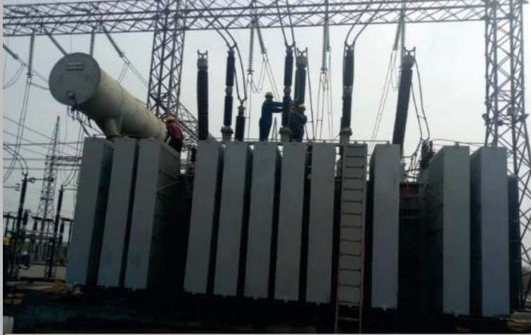
300MVA power transformer in Asaba Transmission Substation, Delta State, commissioned Friday, 10th January, 2020
