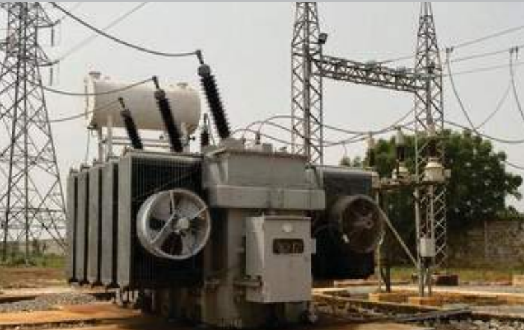
30MVA Power Transformer in Egbin Transmission Substation, Lagos State, commissioned Thursday, 23rd January, 2020
