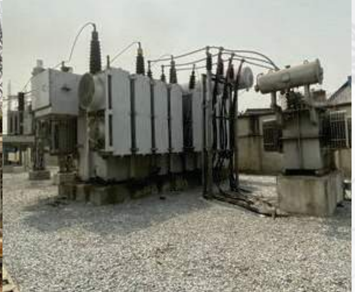
45MVA 132/33kV power transformer in Apapa 132/33kV Transmission Substation, Lagos State
