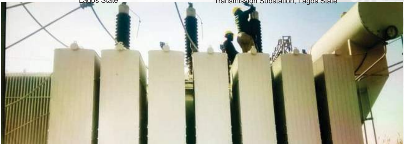
60MVA 132/33kV power transformer in Gusau Transmission Substation, Zamfara State
