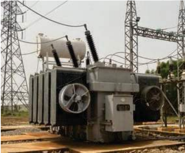
30MVA Power Transformer in Egbin Transmission Substation, Lagos State
