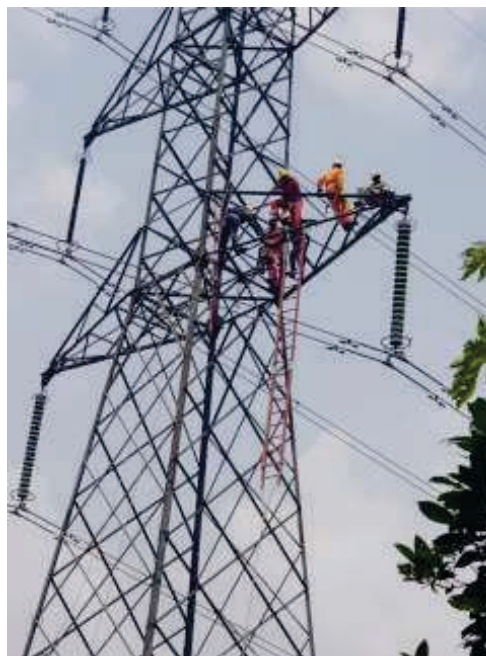
TCN engineers replacing insulators
