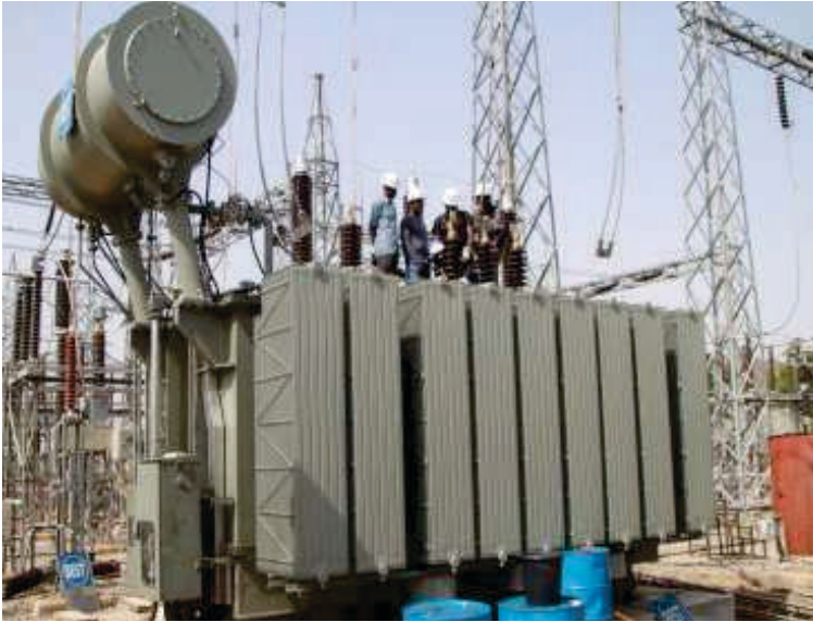
The brand new 60MVA transformer
