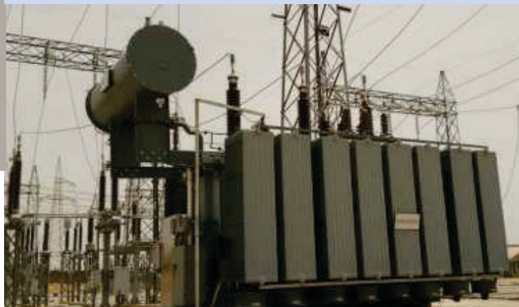
The new 40MVA transformer
