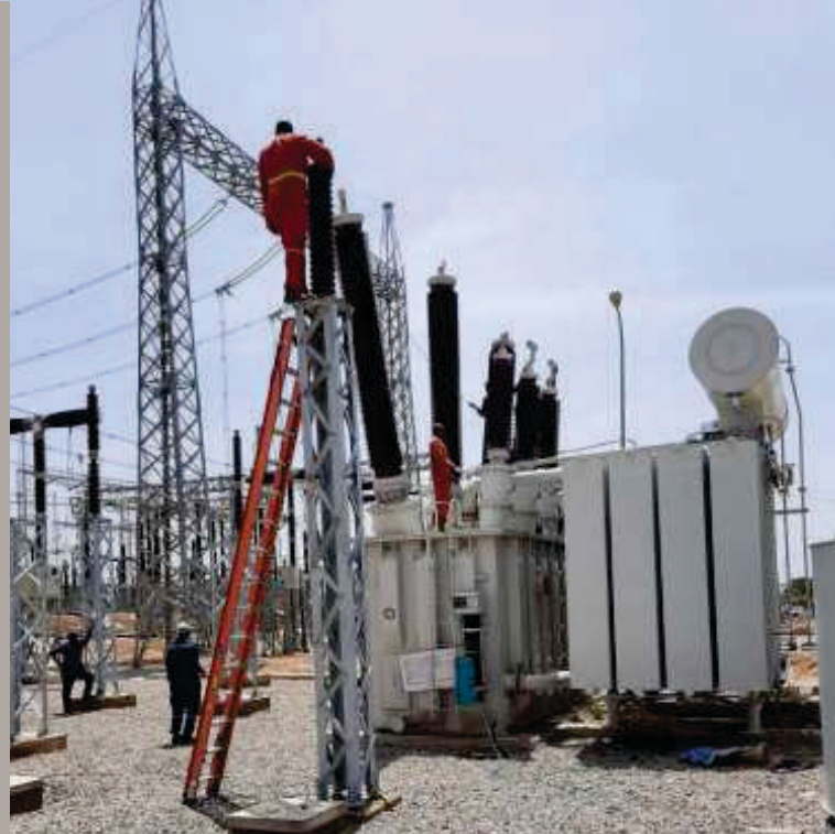
The new 330kV reactor
