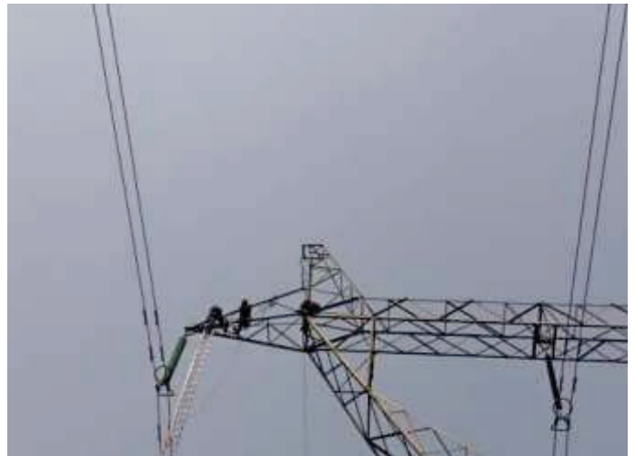
Replacement of corroded glass disc insulators on Tower number 425 at Ikeja West - Osogbo 330kV line.
