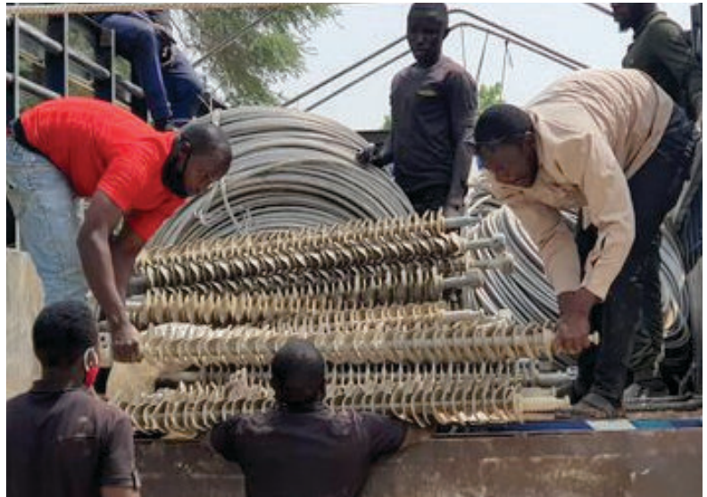
Offloading of insulators and cables
