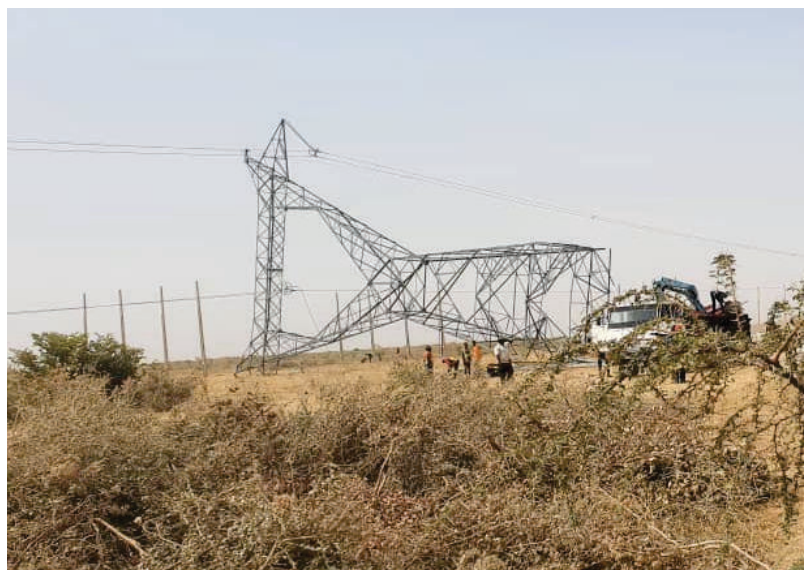
One of the damaged towers
