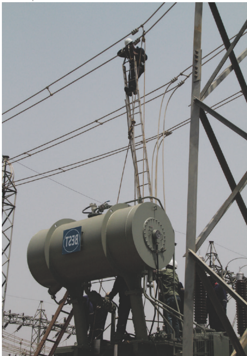
TCN engineers installing the new 60MVA power transformer at Kubwa Substation
