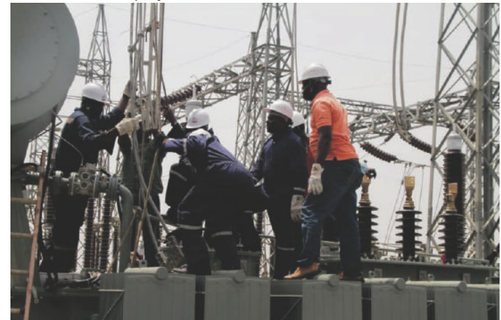
ED TCN-TSP, Engr. Victor Adewunmi, accompanied by some TCN engineers visited Kubwa 2x60MVA 132/33kV Transmission Substation, Abuja, to inspect on-going installation of a brand new 60MVA transformer by TCN in-house engineers.
